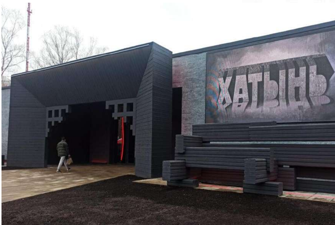
Reconstruction of the Khatyn State Memorial Complex
