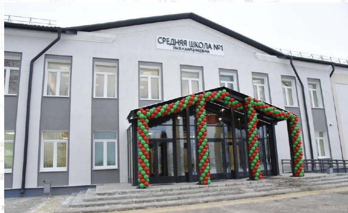
Reconstruction of the building of the State Educational Institution "Secondary School No. 1 named after V.N. Martsinkevich, Krupki"
