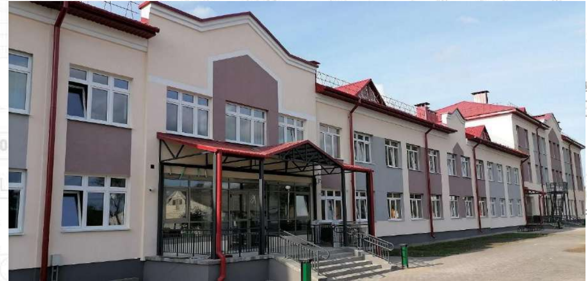
Reconstruction of a school building into a kindergarten-secondary school educational and pedagogical complex in the village of Pervomaysky, Lida District
