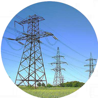
Specialized works (wiring, thermal insulation, commissioning, technic works and etc.)
