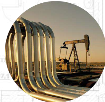
Installation of technological equipment and pipelines
