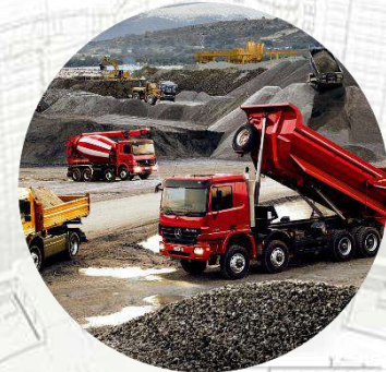
Providing specialized construction and lifting equipment
